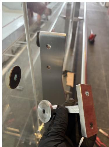
Stainless base plate - after restoration
