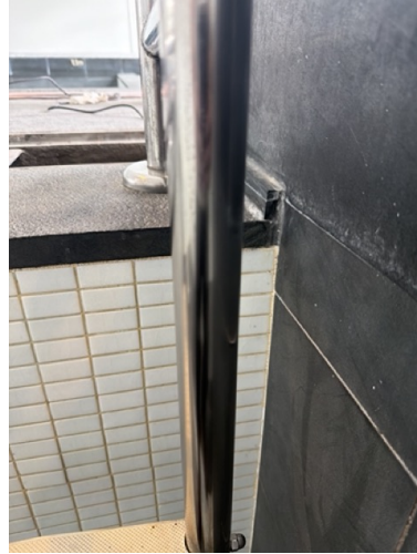
Bracket / glass fitting assembly - after restoration
