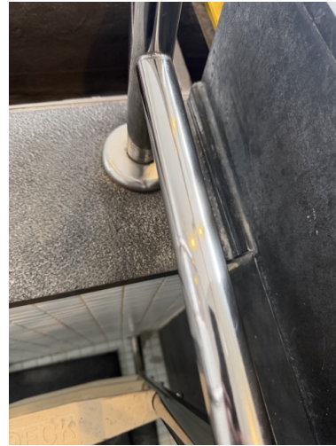
Handrail surface - after restoration
