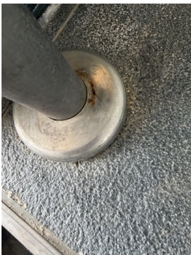
Stainless post / handrail section - before restoration
