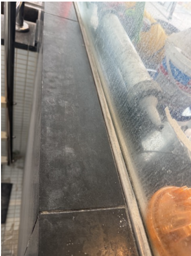
Stainless trim / channel adjacent to glazing - before restoration
