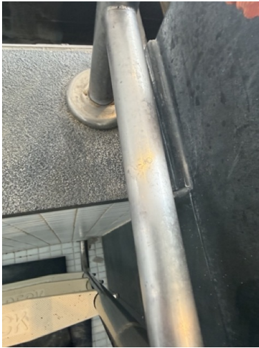
Handrail surface - before restoration
