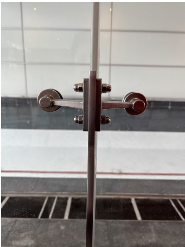
Additional completed stainless fitting detail
