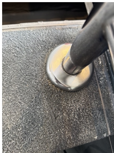
Stainless post / handrail section - after restoration
