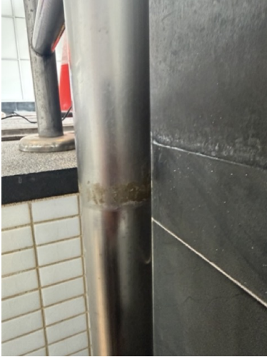
Bracket / glass fitting assembly - before restoration
