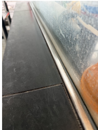
Stainless trim / channel adjacent to glazing - after restoration
